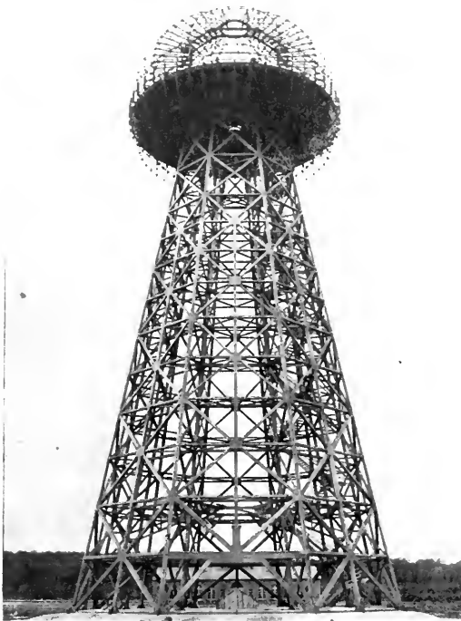
FIG. 2.—TESLA CENTRAL POWER PLANT AND TRANSMITTING TOWER FOR WORLD TELEGRAPHY, WARDENCLYFFE, LONG ISLAND, N. Y.
